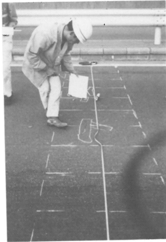
Figure 3 Sketching of cracks at site
