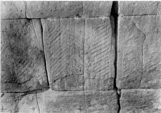
figure 2: natural stones with different level of weathering
