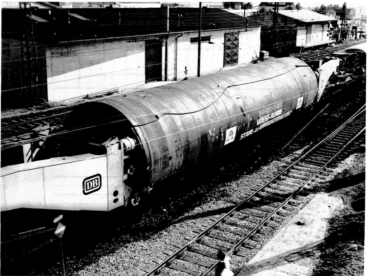
Fig. 6: Special transport of a chemical reactor for the oil industry (Photo Austrian Federal Railways)
