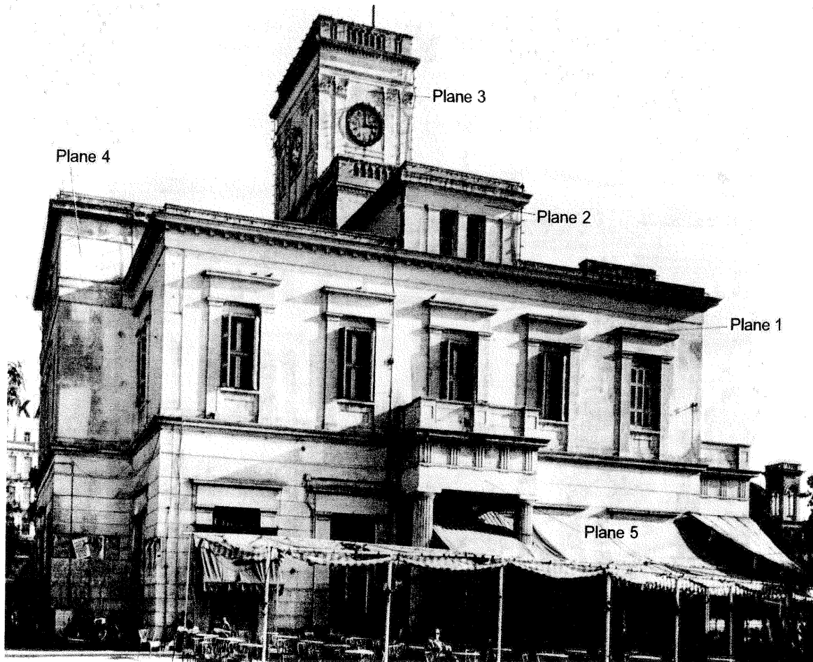
Fig. 2 Photograph of the western side of the building
