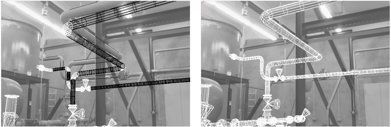
Figure 6: Orientation of image using visible pipe-edges and known position of pipe-segments
