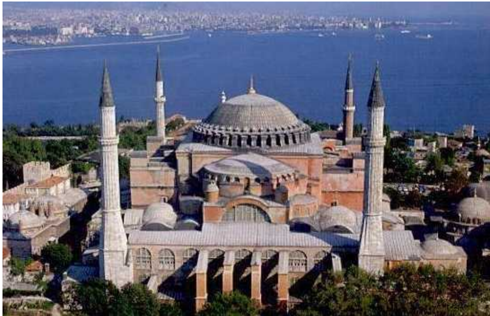
Figure 1. A general view of Hagia Sophia
