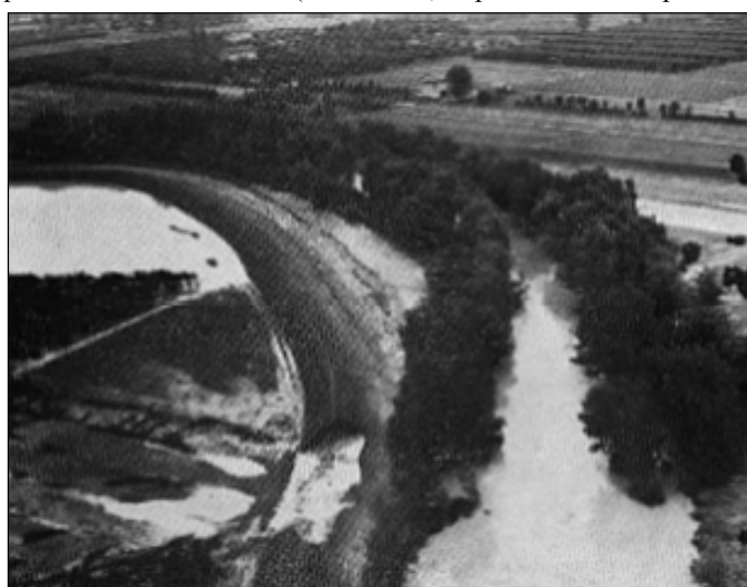
Figure 3. Breach in the embankments of the Panaro river in occasion of the flood occurred on 25-09-1973 (Moratti & Pellegrini, 1977).
