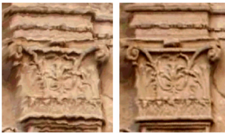
Figure 4. Projection of the image on an original 3D model (left). Projection of the image on a 3D model depurated of the disturbance (right).
