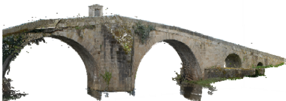
Figure 6. Coloured point cloud of Carracedo Bridge.
