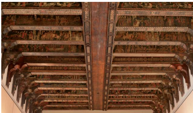
Figure 3. The wooden ceiling of the “Magna” Hall.
