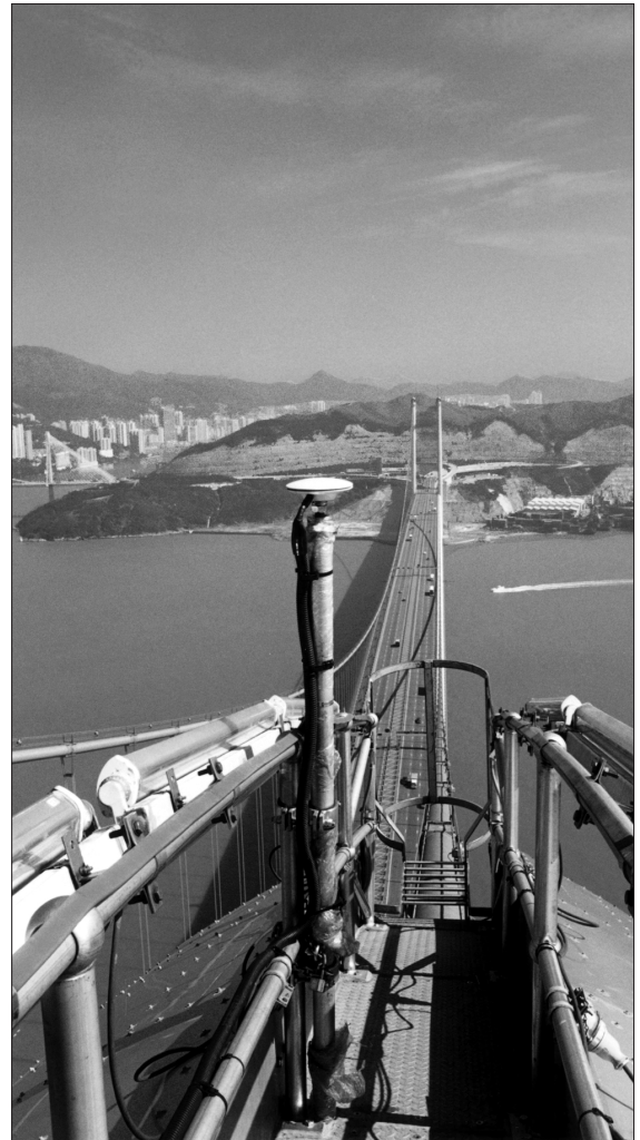
All bridges to the new Hong Kong airport are monitored using 29 GPS sensors from Leica Geosystems. Monitoring the environment and large structures is one of the fast growing areas in which Leica Geosystems wants to become a leader.
