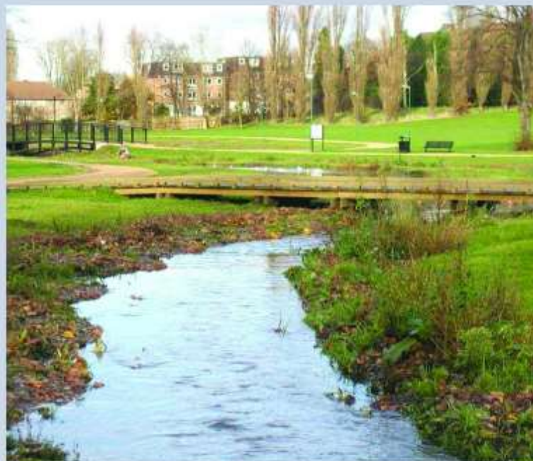
Culverted watercourse replaced with natural meandering watercourse
