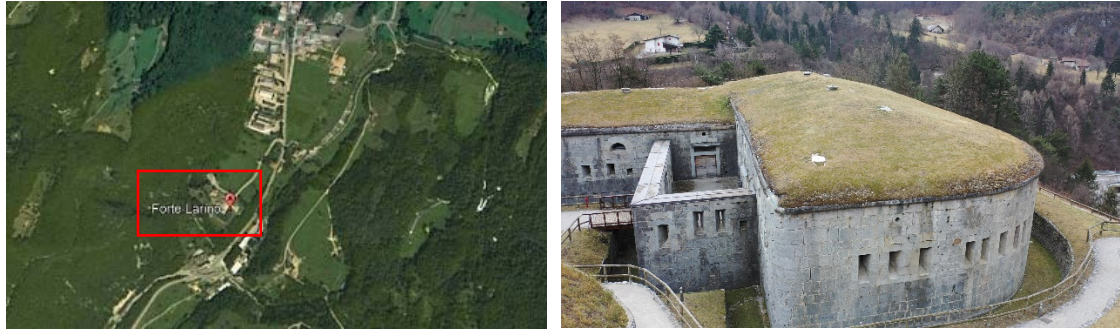
Figure 3: The UAV-based dataset of the WWI Larino Fort (Lardaro, Italy) used for the evaluation of PhotoMatch. The entire area (left) and an oblique UAV image used for testing the tool (right).
