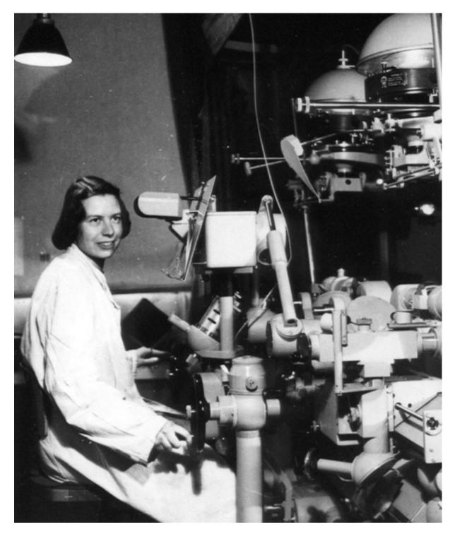
Aino is shown here doing work on the Zeiss Planigraph.
