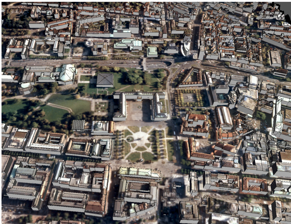
Figure 8: Visualization of reconstructed buildings with aerial image overlaid
