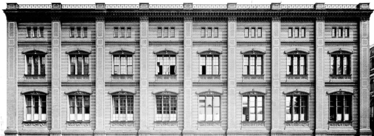
Figure 4: Rectification result of the “Bauakademie”, based on geometric information provided in historical data (rectification scale 1:50)
