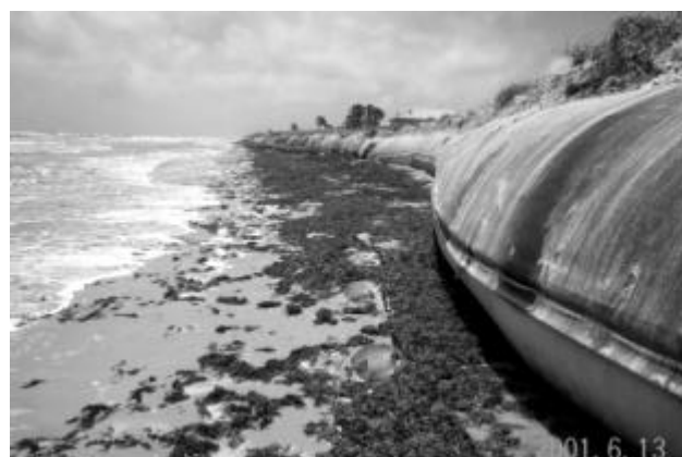
Figure 12. Geotube installed in front of the beach scarp at Bolivar Peninsula during July 2001
