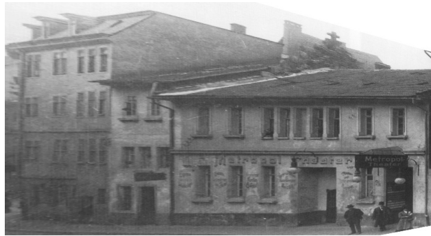
Fig. 12: Rectified view of the image shown in Fig. 2.
