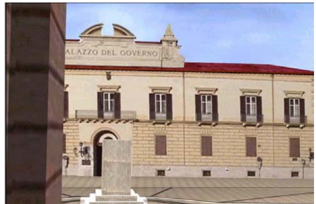
Figure 8. View of the Province Palace from the portico
