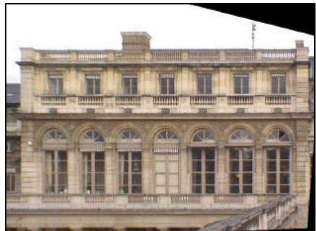
Fig 4. Rectified Image of a frontage of the Palais Royal
