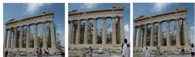
Figure 7. Photographing of Parthenon (east elevation)
