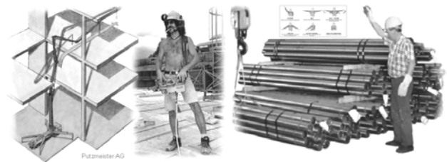
Figure 2. Machine drivers work without visual contact and with help of briefing persons (Source left: Putzmeister AG).
