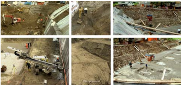
Figure 13. Excavations are special earth body forms - geometrically defined and quasi interiors (Source: Internet).
