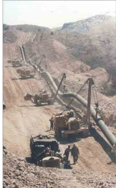
Figure 1. Pipeline construction at hilly area ( http://osfm.fire.ca.gov/gishead.html )
