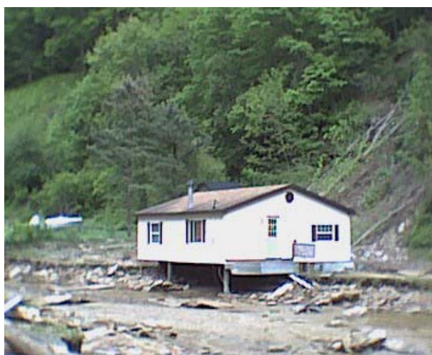
Figure 3. Residential home with eroded foundation
