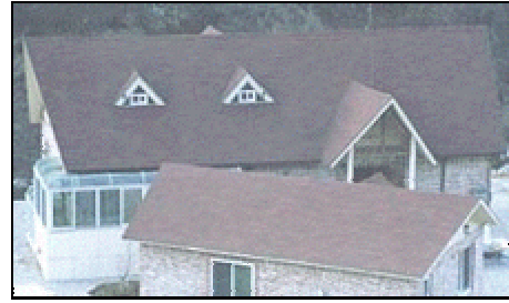
Figure 5. 'Asphalt Shingle' as Roof Material
