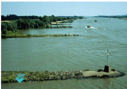
Figure 3. Groynes along a Dutch river.
