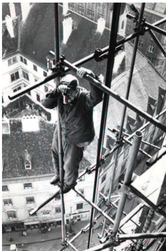
Foramitti at dangerous recording work high up on a scaffold (St.Stephen, Vienna 1960)
