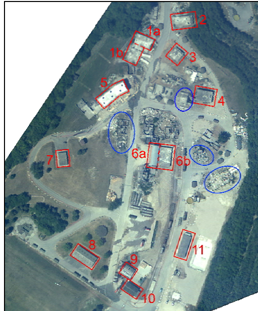
Figure 1: Aerial image of the test area (in red: undamaged buildings, pancake collapses, inclined planes; in blue: heaps of debris, outspread multi layer collapse)
