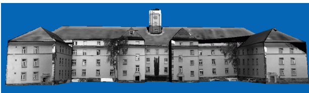
Figure 13. Textured building surfaces (north view)
