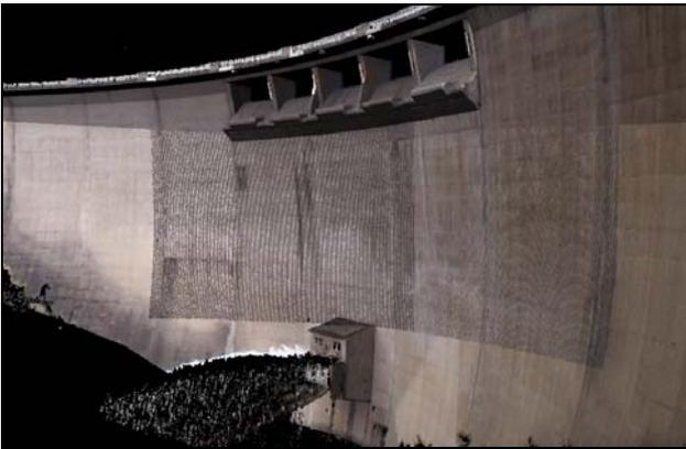
Figure 5. Global laser scan model applied to the whole dam structure.
