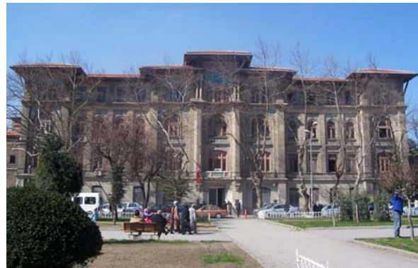
Figure 1: The pre-cleaned situation of the front façade
