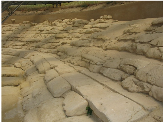
Figure 5. The Koilon of theatre of Eraclea Minoa after the restoration
