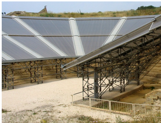
Figure 6. Today the Theatre is protected temporarily by a cover
