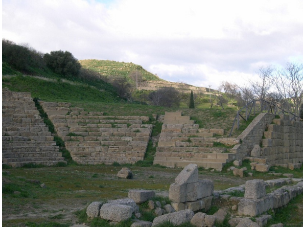
Figure 8. The Koilon of Morgantina's theatre before the last restoration
