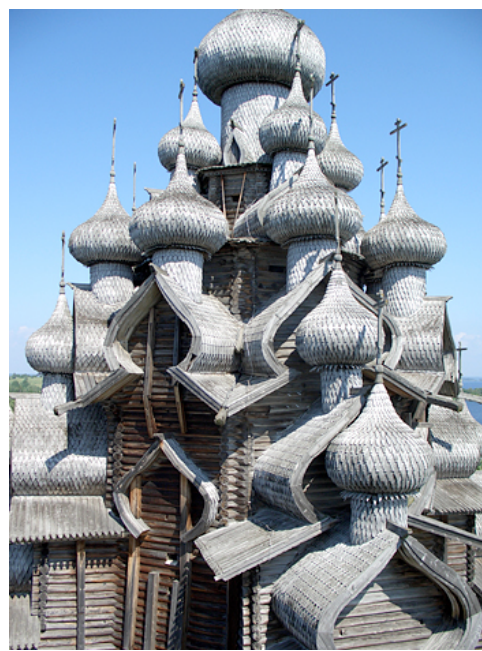
Figure 2. The domes of the Church of Transfiguration.
