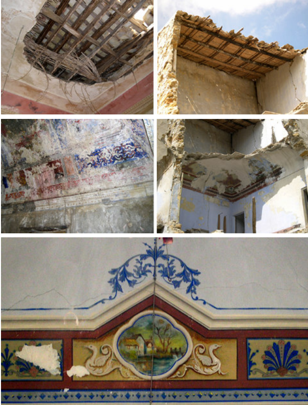
Figure 7 – 8. Some example of roofings and some example of internal plaster.
