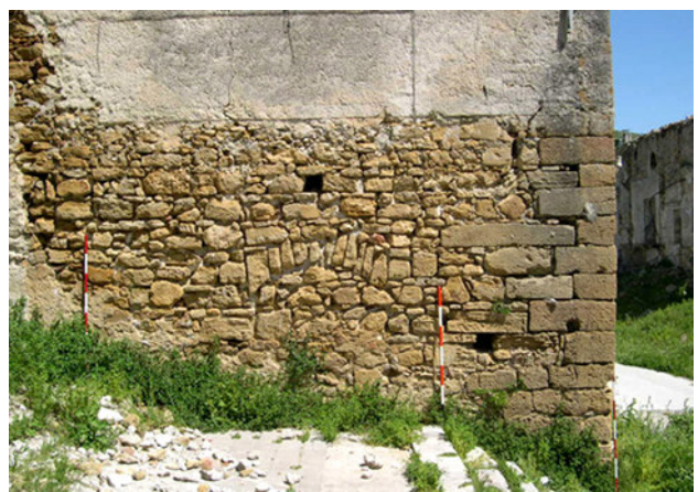
Figure 6. Building's edges made of large dimensioned squared rocking.
