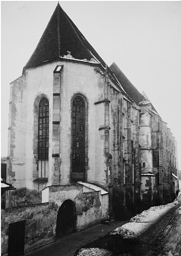
Figure 1. The Church before the conservation works in 1958
