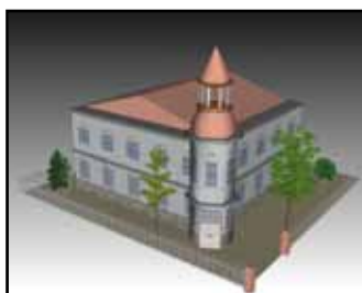
Hachinohe police station
