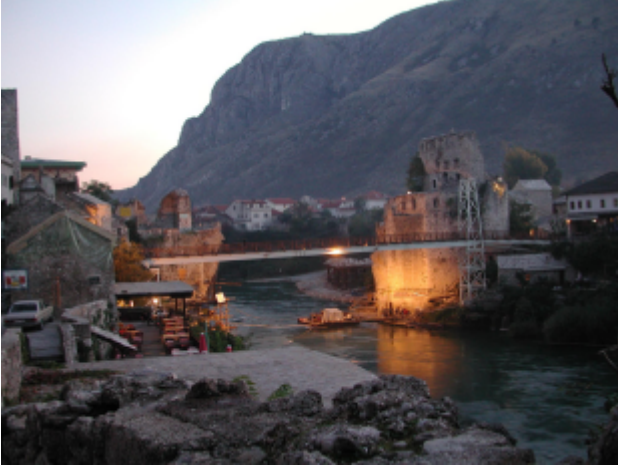
Figure 2. The figure shows the Mostar Bridge some time after the Bosnian War. A temporary bridge was put in place. The bridge has recently been restored and reopened.
