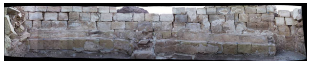
Figure 8. An interior panoramic image of a wall of an apse. The images are rectified onto cylinder. This sequence of five concentric images corresponds to an approximate angle of view of 40^\circ \times 210^\circ .
