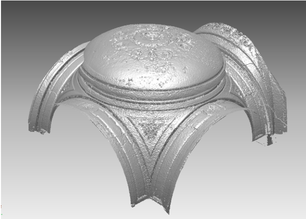
Figure 5: Laser scanner surface of a part of the vault of the Villa Reale entrance. The represented surface is the meshed original surface. The resolution is about 0.5 cm and this let to model with good accuracy detail whose dimension is bigger than 2- 2.5 cm.
