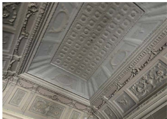
Figure 19 An example of the 3D model of the "Pendola room" in the Villa. In the upper image the meshed surface of the vault is assembled on the 3D textured model of the walls. Below the same model but with the colour orthophoto projected onto the vault.
