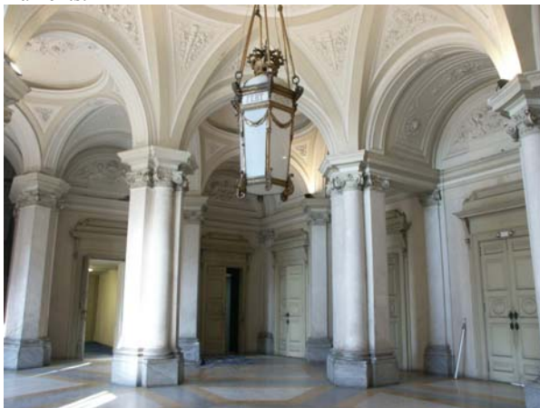
Figure 2. View of the entrance hall before the restoration work. It's possible to see the complex geometry of the vaults: almost vertical elements, many undercuts, the diffuse light color and the lack of texture on the vault doesn't let a good matching in the 3D model generation in particular when taken are very close to the vaults.
