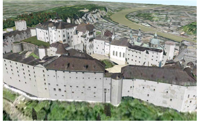
Figure 3. The Fortress Hohensalzburg in Salzburg, Austria. The building is part of a area-wide 3D city model which was generated by CyberCity. The geometry has been extracted from stereo aerial images using photogrammetry. Roof and facades have been textured semi-automatically using oblique aerial images. © CyberCity AG, ViewTec AG, Forest Mapping Management GmbH
