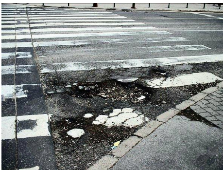
Figure 1. Potholes and cracks on the pavement
