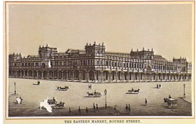
Figure 4. Eastern Market, Bourke Street Melbourne, ca. 1888 Source: State Library of Victoria http://www.statelibrary.vic.gov.au
