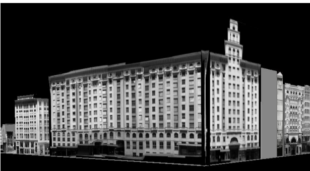
Figure 16. Detail of the Temperance and General building, situated at the north-east corner of the study area
