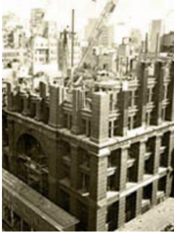
Figure 6. Colonial Mutual Life Building Demolition, 1960. Museum of Victoria. http://www.museum.vic.gov.au/colonial/demolition.asp
