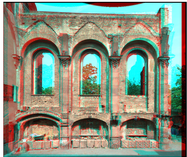
Figure 3. Stereoscopic view of a panoramic image pair (Dresden Trinitatis church, EYESCAN M3D, c_k 35 mm. RGB CCD-line with 10.000 pixels)
