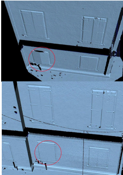
Figure 7: Change of geometric position of some elements along the facades of the villa between different scan epochs led to a registration failure.
