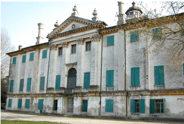
Figure 2: View of the north facade of Villa Giovanelli
