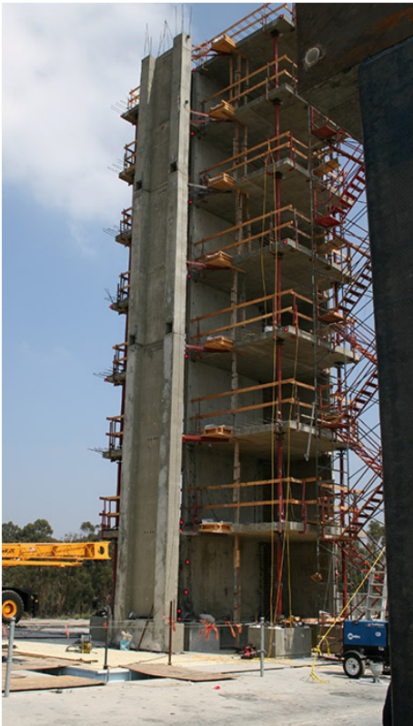
Figure 5. Building with target arrays powered on
