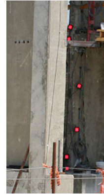
Figure 6. Close up view of adaptive target arrays powered on
