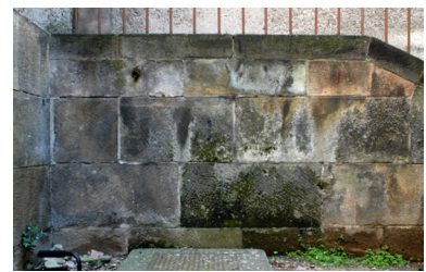
Figure 9. Damaged sand stone wall, overview image taken with digital camera.
