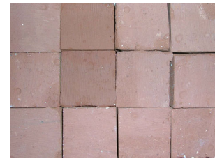
Figure 5. Wall consisting of small bricks, two of the bricks are moist. The photo was taken with a digital camera.
