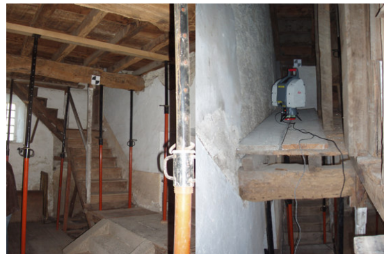
Figure 4. Interior part of the retable. Laser scanner Cyrax 3000 in a complex area.
