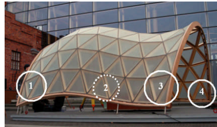
Figure 2. The dimensions of four corner triangles of the pavilion were measured in order to get approximate scale for the photogrammetric model.
