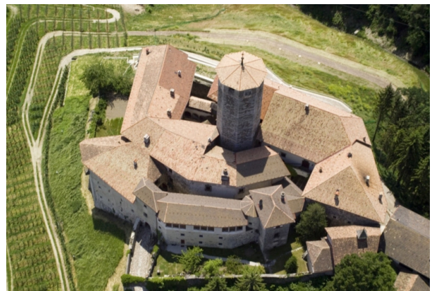
Figure 14: An aerial view of the Valer Castle, located near Trento, Italy. This is a typical example of architecture containing streets and courtyard very narrow and quite complex for successful and precise 3D modeling.
