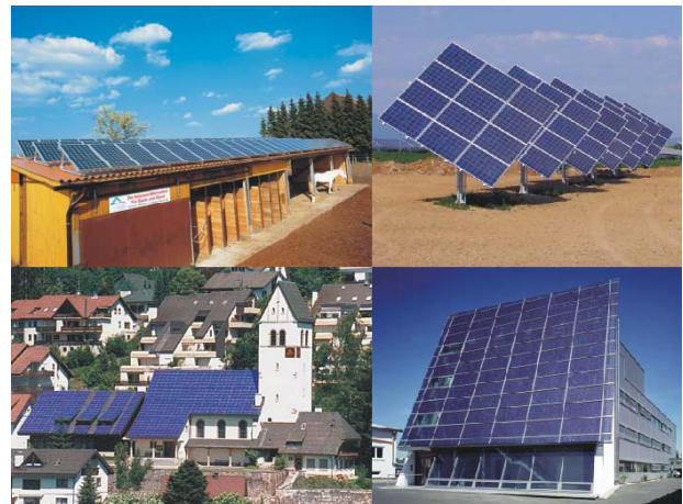
Figure 2. Ground-mounted and building-integrated photovoltaic arrays
